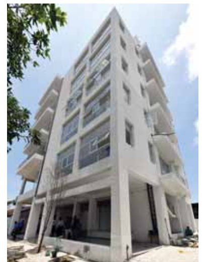
New Head Office Complex in Narahenpita
